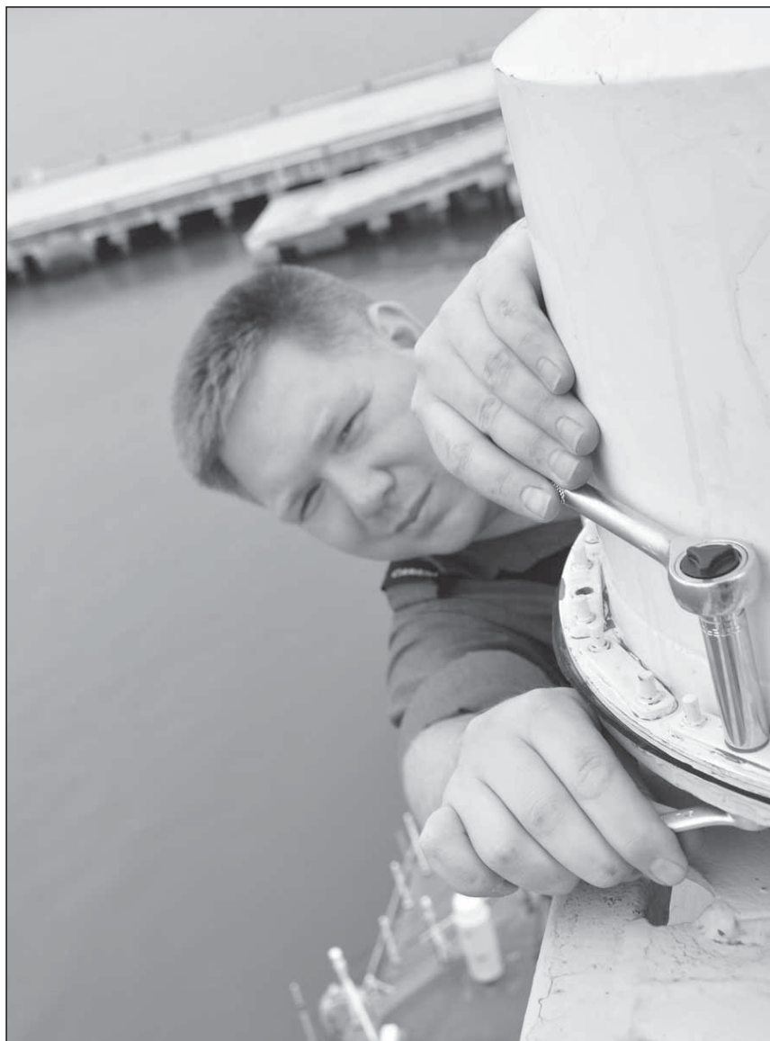
Photo courtesy of HMCS Winnipeg PO2 Kirk Kendall performs maintenance up high on HMCS Winnipeg's main mast.
