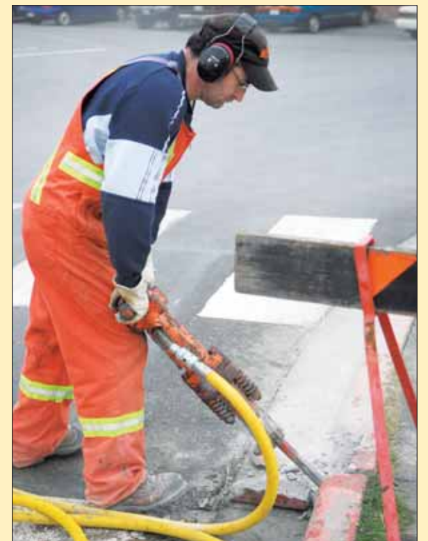
Base Construction Engineering employees keep CFB Esquimalt in tip top shape, performing maintenance and repairs ranging from painting to roadwork.
