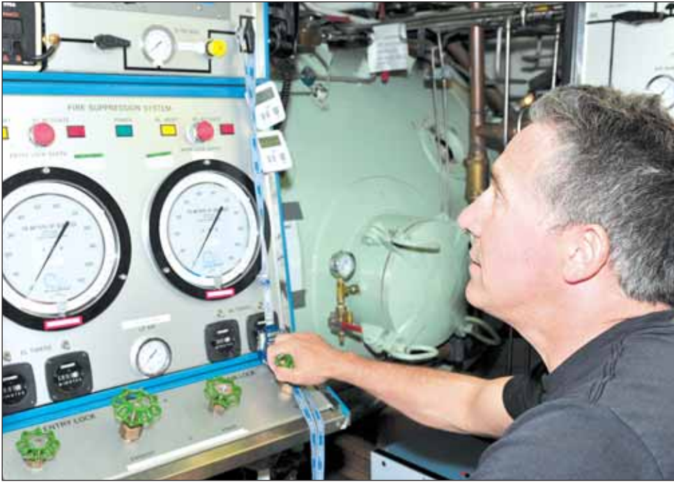
Above: PO2 Rob Majore adjusts the amount of gasses entering the recompression chamber for a diver who has just come out of the water. To get comfortable with the process of recompression, divers simulate time in the recompression chamber following each dive.
