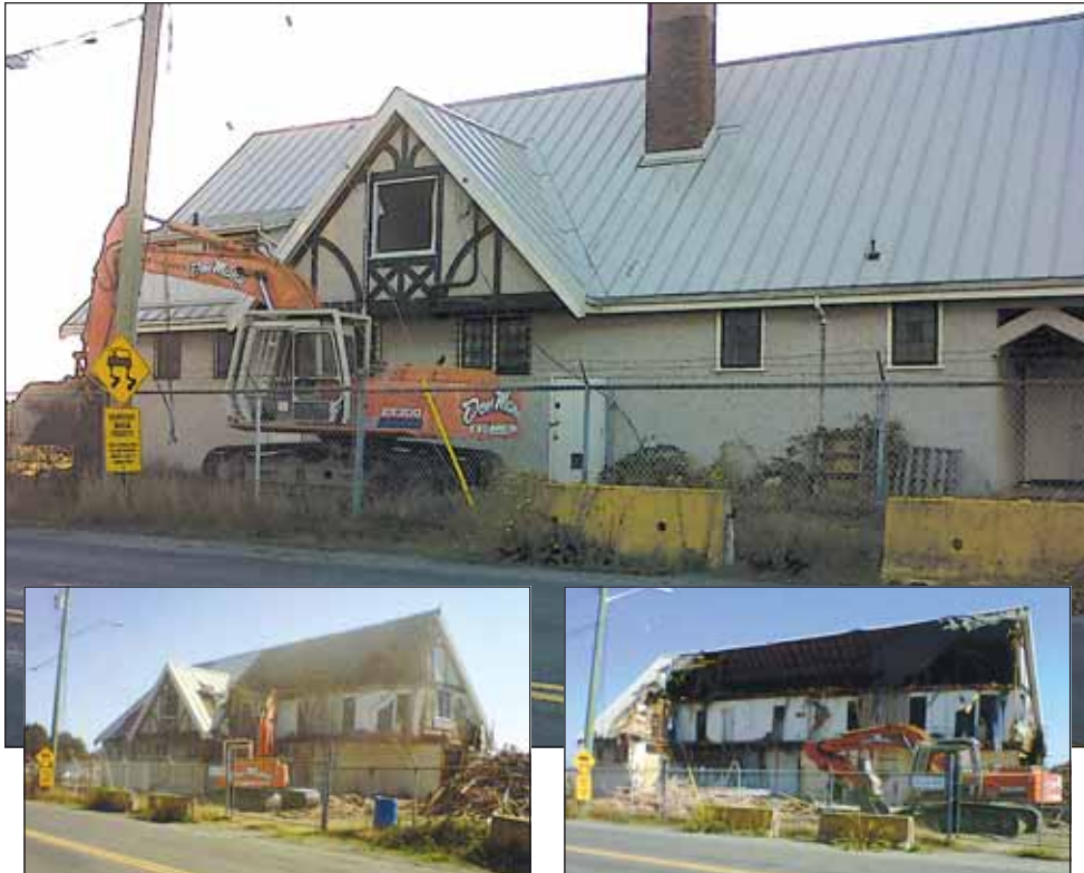
Base Construction Engineering has removed this building, which served as a pub, married quarters, and degaussing station at one time in its long life near Esquimalt Lagoon.
