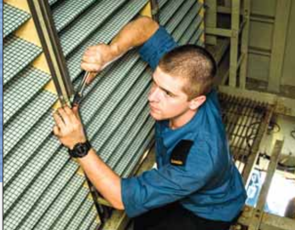
OS Keagan Harder conducts filter maintenance in the general turbine inlet.
