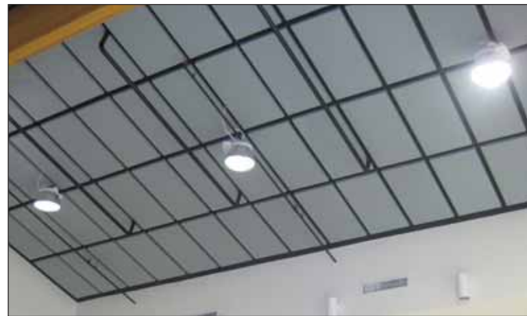
Above: Energy efficient LED lights are now installed in the Colwood Pacific Activity Centre.
