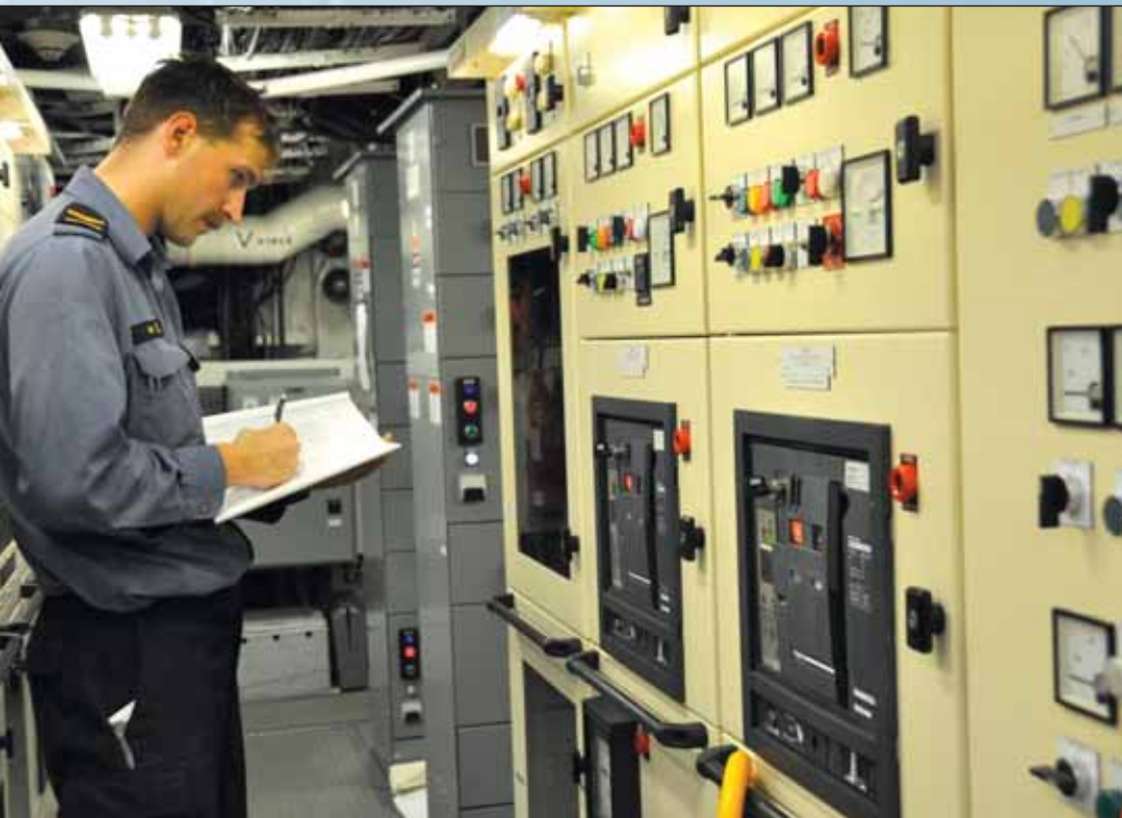
Master Seaman Kyle Uhlig, a Marine Engineering System Operator, conducts his daily rounds in the Main Switchboard Room in HMCS Brandon while deployed to the eastern Pacific on Operation Caribbe.
