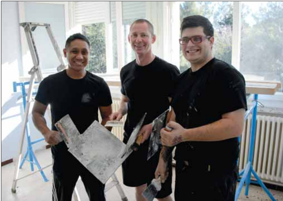
Photos by Slt Jamie Tobin, HMCS Winnipeg LS Jose Villano, LS Andrew Drake and AS Matthew White from HMCS Winnipeg help with renovations at the Résidence solidaire les Favières in Toulon, France, during a break from Operation Reassurance Nov. 18.
