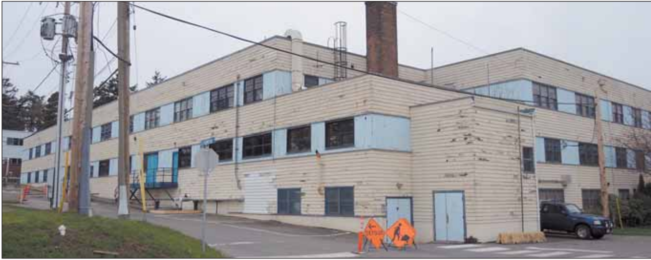
A view of Dockyard Building 11 from the intersection of Plumstead Street and Dockyard Road south. DY11 and its neighbouring DY29 were built in the 1940s but are currently being prepared for demolition.
