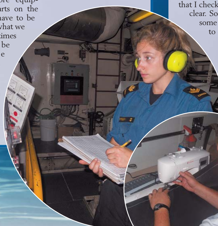
A Marine Technician records information from one of the ship's diesel alternators as part of rounds.
