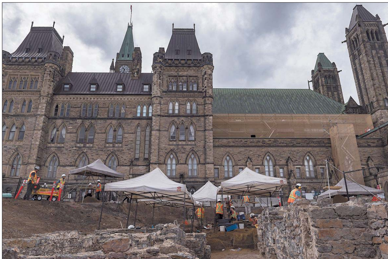
The foundation walls of a 19th-century guard house beside the East Block building on Parliament Hill are excavated as part of the assessment work for the estimated 10-year rehabilitation of the Parliament Buildings in Ottawa, Ontario, on July 30. Photo by Able Seaman Camden Scott, Army Public Affairs
