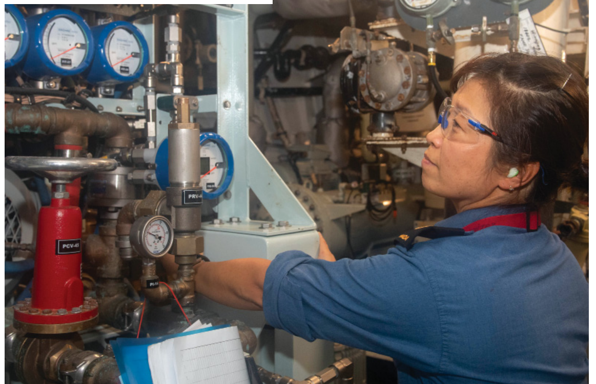
S2 Hyang Mi Bae conducts rounds on the starboard Shipboard Reverse Osmosis Desalinator.
