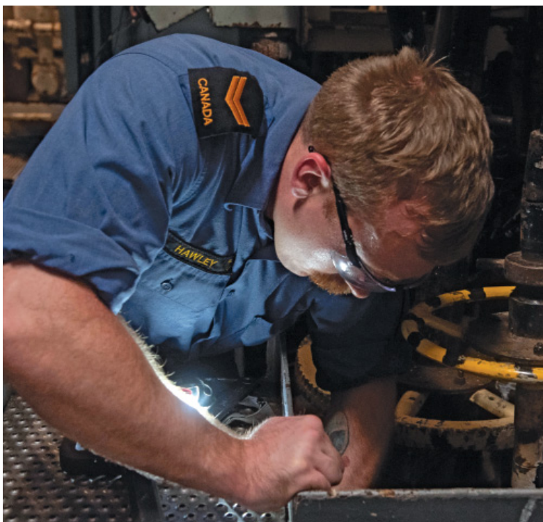
S1 Sheldon Hawley conducts maintenance on valves in the Forward Auxiliary Machine Room.
