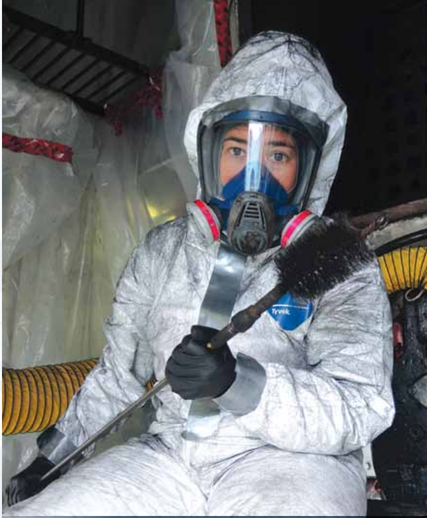
Dyan Day uses a giant metal pipe cleaner to remove oxides and soot from the Scotch Marine fire tube boiler aboard YD 250.
