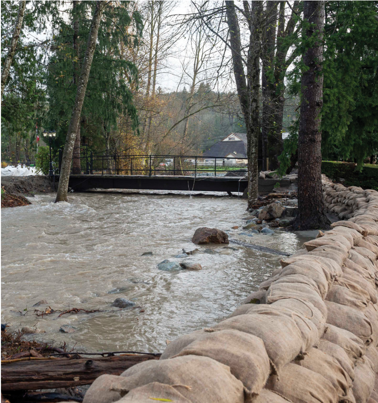
Members of Lord Strathcona's Horse (Royal Canadians) Regiment built a wall on Nov. 24 to protect homes from potential flooding. After heavy rain a few days later, the wall accomplished its purpose in Abbotsford. Photo by MCpl Nicolas Alonso, Canadian Forces Combat Camera, Canadian Armed Forces Photo
