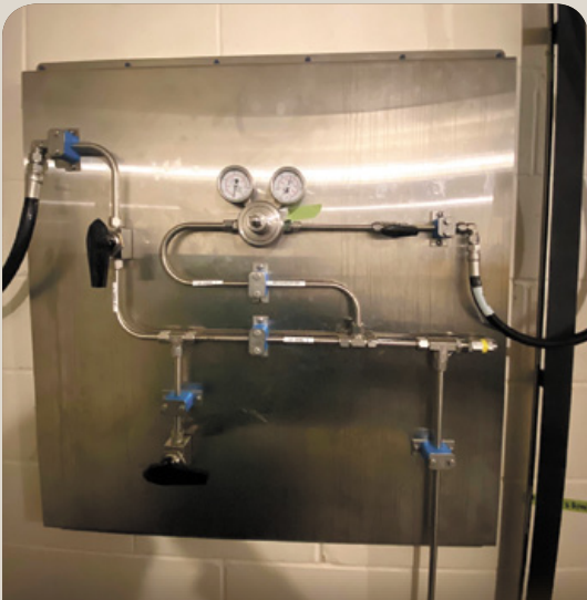
A main control panel supporting a newly assembled clean air system.
